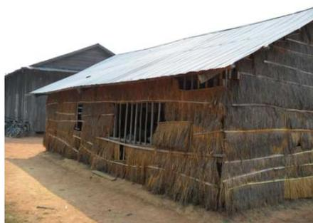
Instable walls made of clay and straw
