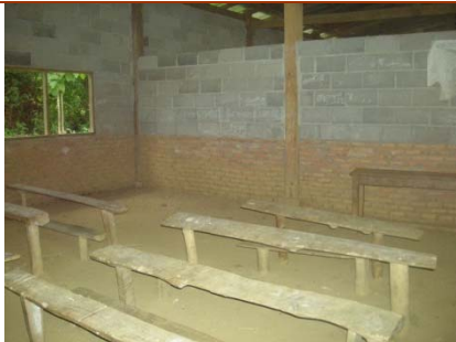
Inside the partly existing structure
