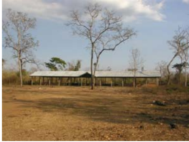
The unfinished school building
