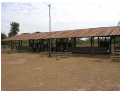
The existing school building will be replaced
