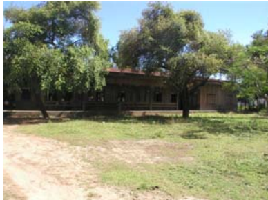
The nursery school needs renovation
