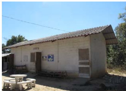
The existing boarding house for 52 students
