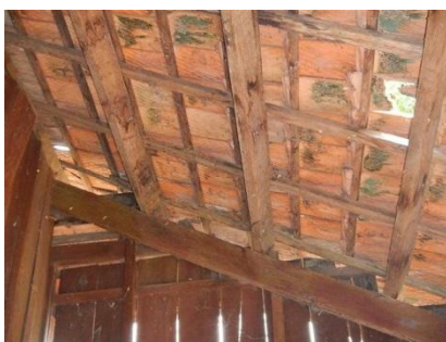
The current state of the roof
