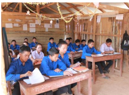
Crowded classrooms with dirt floors in a rotten building
