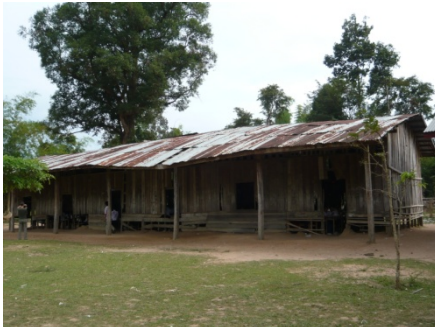
An old building from the outside...
