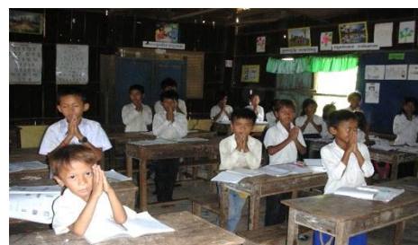
Primary students of Ta Pon Primary School in their rotten and unsafe building
