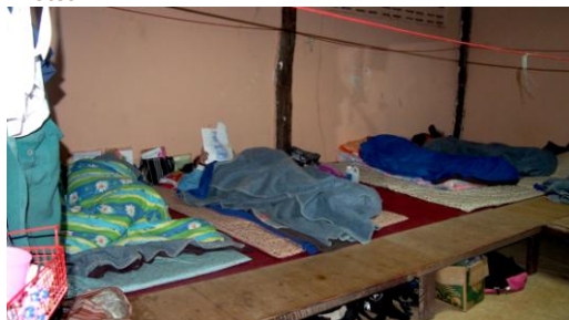
The boarding house is overcrowded and in disrepair
