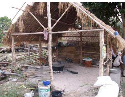
View into the current school kitchen
