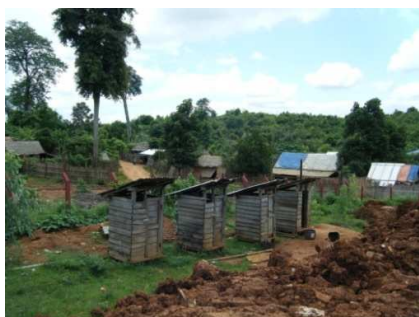
Toilet facilities to be replaced.
