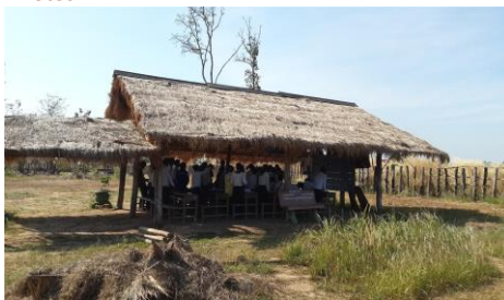
1 st building made from wood and grass leaves. Students are exposed to wind and rain
