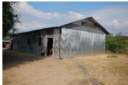
The temporary school building made out of zinc
