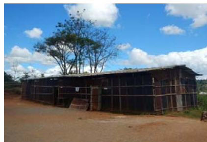
This wooden building is not only more prone to degradation, but also does little to protect students against the natural elements
