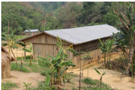
Nam Duan Lower Secondary School compound
