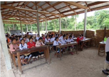
Some classes are taught in incomplete buildings
