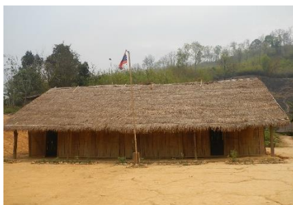
Temporary building erected by the community
