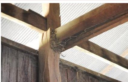
Some columns are infested by termites and are close from collapsing
