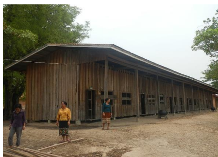
The old school building was last repaired in 1996
