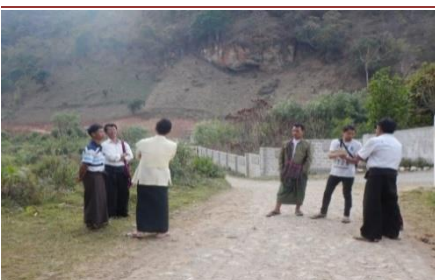
Searching for a good location to build the boarding house. Not easy because of the soft land and nearby mountains.
