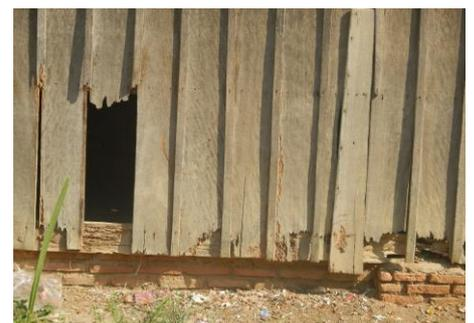
The slat walls are infested by termites and on the verge of collapsing.
