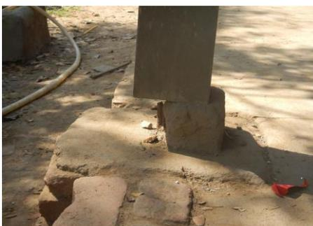
The building is supported by substandard wooden columns bolted on concrete piers.
