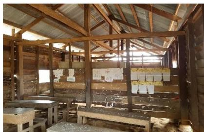
The zinc roof causes the temperature to increase during the hot season and it is very noisy when it rains.
