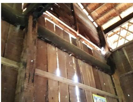
The roof, the wooden walls and beams perforated by moisture and vermin. The foundation is unstable and very scary for the students, their parents and teachers.
