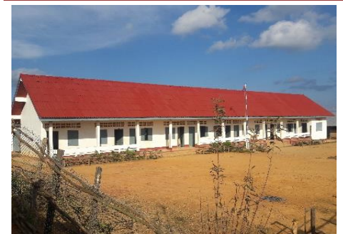
The recently-built concrete building 100% supported by the Laotian government. The classrooms are now seriously overcrowded.
