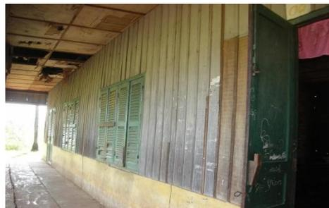
The battered ceiling of the wooden buildings with its run-down, unhygienic grounds and broken doors and windows.
