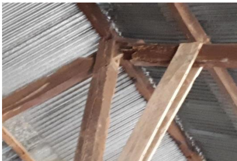
The wooden beams are infested with termites and the roof can collapse anytime, potentially hurting children in class.
