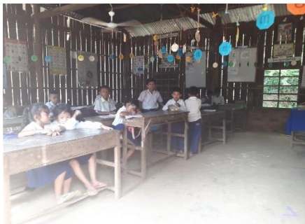
Primary students attending class in one of the rotten wooden buildings
