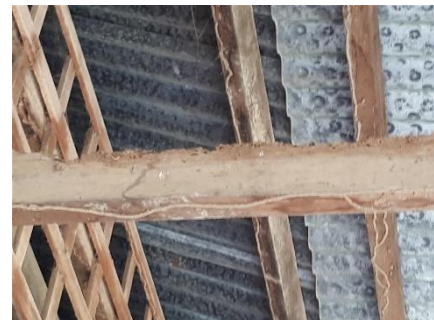
The wooden beams are infested with termites and the roof can collapse anytime, potentially hurting children in class.
