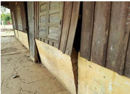
The two wooden structures have severely deteriorated and are on the verge of collapsing, endangering children attending classes.
