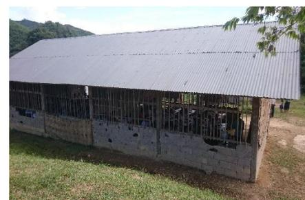
The rear view of the dilapidated building B. The unfinished cinder block walls are severely corroded.
