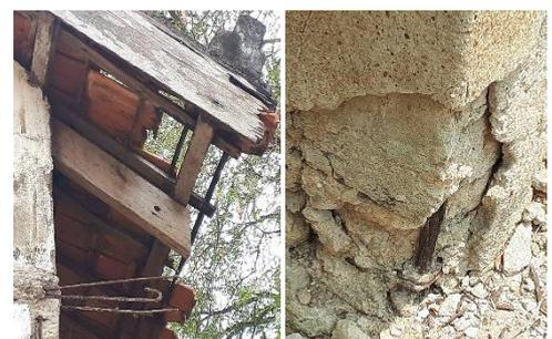
The structures have reached the near collapse limit stage, endangering the school children. The reinforcement bars are corroded and rusted. The concrete walls are heavily cracked and the wooden roof shingles are also decaying. A replacement of the building is urgently needed.
