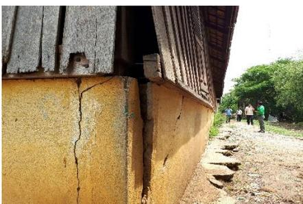
The wooden columns and walls have deteriorated notably and are on the verge of collapsing, endangering children attending classes.
