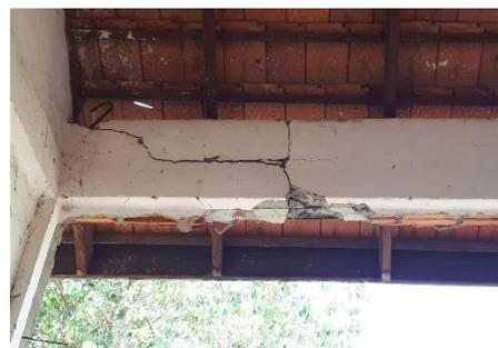
The horizontal beams and walls are severely cracked and are on the verge of collapsing; endangering children attending classes.
