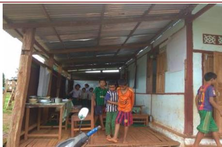
The construction is mainly made out of zinc metal sheets and the interior became unbearably hot during the hot season and frigidly cold during the cold season.
