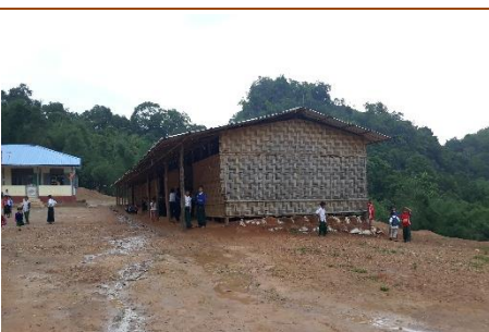
The interior become unbearably hot during hot season and the dirt floor turns muddy during the rainy season.
