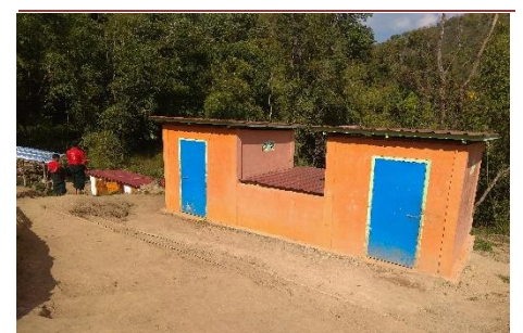
The existing 6 toilets at the back of the school are not enough for 190 students and 9 teachers.
