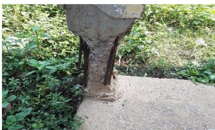
The reinforcement bars have become rusted and the supporting pillars are deteriorating quickly.
