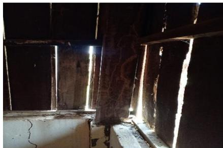
The concrete base walls are heavily cracked and in an advanced state of decay and the wood slat walls are infested by termites. The building is structurally unsound and can collapse anytime soon.
