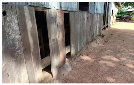
The wood supporting the structure is severely damaged and is on the verge of collapsing, endangering children attending classes.
