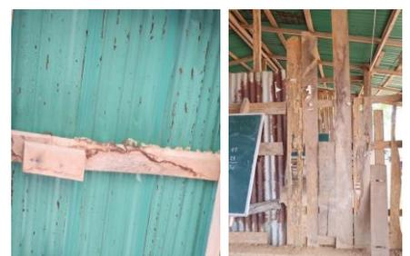
The roof trusses and walls are infested with termites and on the verge of collapsing.
