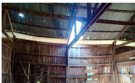
The slat walls and roof trusses are severely damaged by the rain water and termite infestation and can collapse any time, posing a real risk to the children and teachers.
