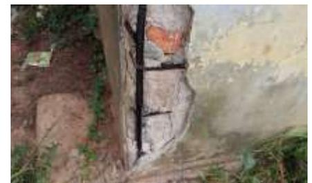
The concrete base wall supporting the structure is severely damaged and is on the verge of collapsing, endangering children attending classes.
