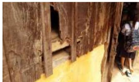
The wooden slat walls and roof trusses are severely damaged by termites.
