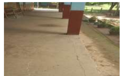
The unfinished concrete floor started to chip and flake off which can lead to severe deterioration overtime. The entire structure became dangerous for the safety of the children.
