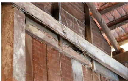
Rotted, deteriorated boards and beams are not only a grim setting for a classroom, but also clear evidence of an extremely unstable, unsafe structure
