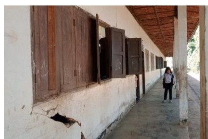
Large structural cracks from the earthquake can be seen on the outside of the building as well as smaller fractures inside the classrooms
