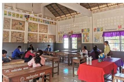
An existing classroom will be renovated to become the new computer laboratory
