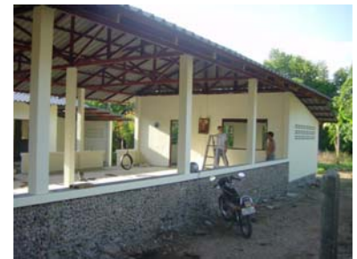
New OPC school is almost finished
