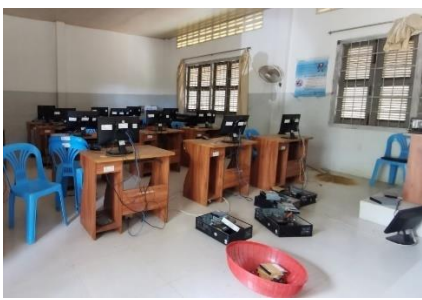
The existing computer laboratory is full of outdated and inoperable computer equipment
