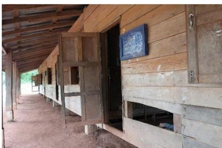
After a decade of use and exposure to harsh Laotian elements, the wooden structure is severely deteriorated and rotting away
