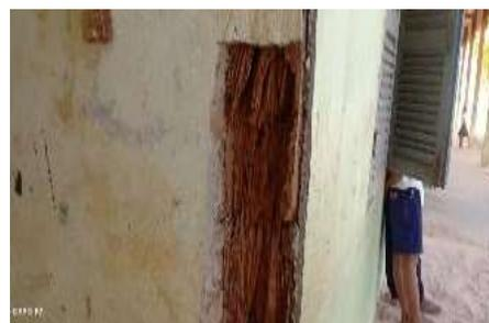
The rotten wood does not offer adequate support
