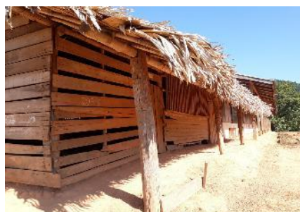
Made of wood, bamboo, and grass, this temporary building is on the verge of collapse.
