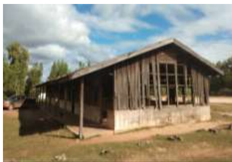
The one classroom building built in 1974 is made of substandard materials, fast deteriorating, and in dire need of replacement
