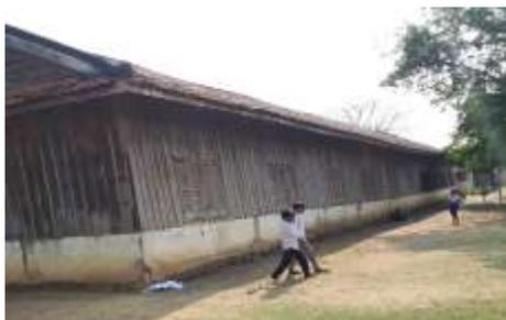
The cracked and friable foundation is close to collapse under the fragile wooden construction.
