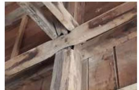
It is only a matter of time before the rotten wood scaffolding collapses.
